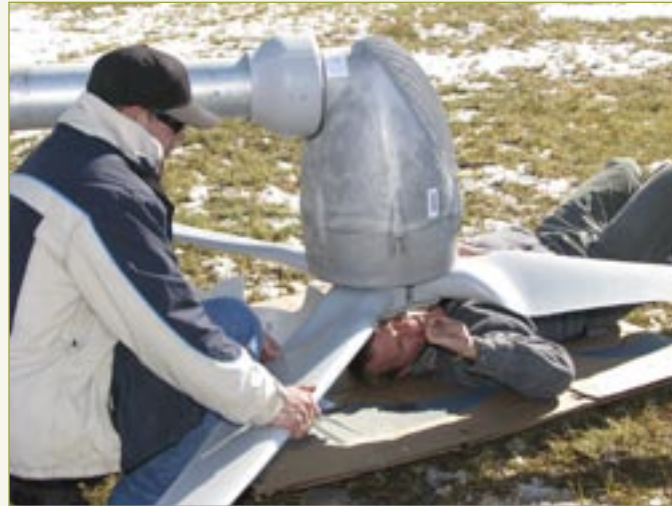
Engineering student Cole Young (left) and Professor Robb Larson adjust wind turbine blades before raising the 50-foot-tall turbine into place. (MSU photo by Michael Becker)
