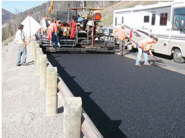
Warm-mix asphalt is placed on Yellowstone's East Entrance Road. The asphalt handled similarly to a conventional mix.
