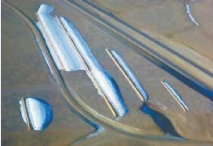
Aerial view shows the snow fence system at Wyoming I-80 Mile 280.8.
