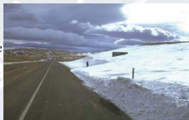
Conditions at Wyoming I-80 Mile 280.8 before the construction of snow fences.
