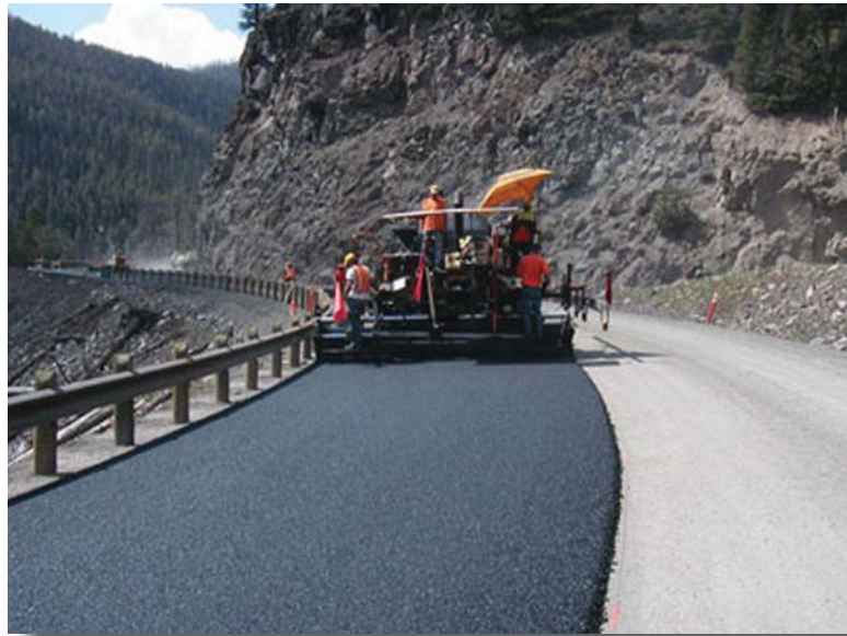
Warm-mix asphalt is placed on Yellowstone's East Entrance Road. The asphalt handled similarly to a conventional mix.
