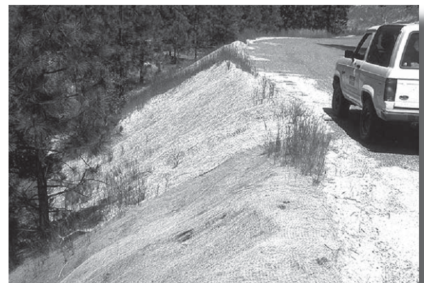
Cover fill slopes, work areas, and other exposed soil areas with straw, netting, rock or other material to protect the ground and promote vegetative growth. Photo & quote from Low-Volume Roads Engineering, BMP Field Guide by Gordon Keller & James Sherar
