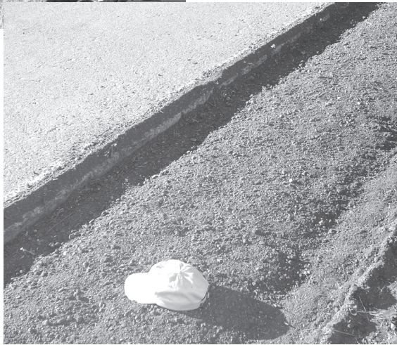
Finished cutout along pavement edge.
