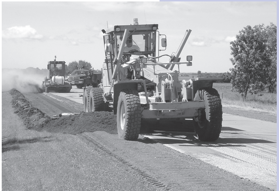
Final shaping of cutout with motor grader
