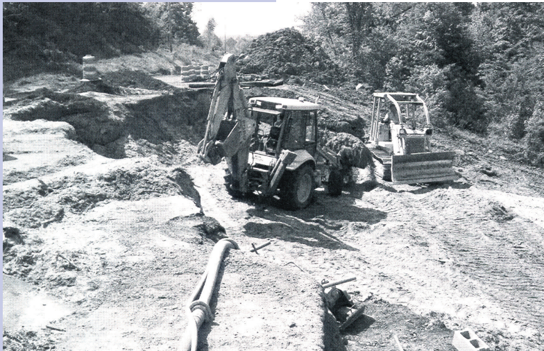
Placing and Compacting Lightweight Sawdust Backfill
