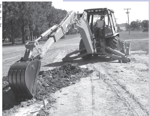
Clay Moore digging trench for classroom exhibit for pipe drainage & surveying
